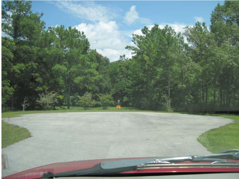
Private road cul-de-sac for subject property facing west
